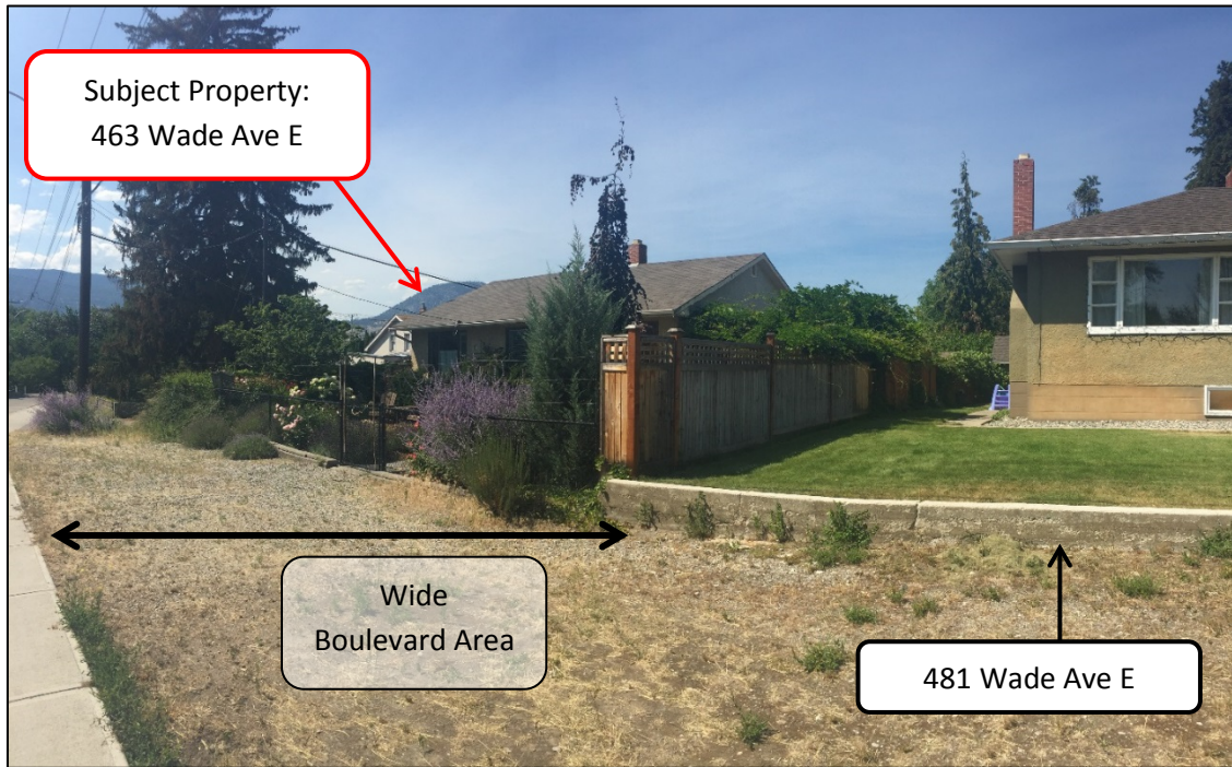
Figure 8 – Looking at 463 Wade Ave E from Wade Ave E
