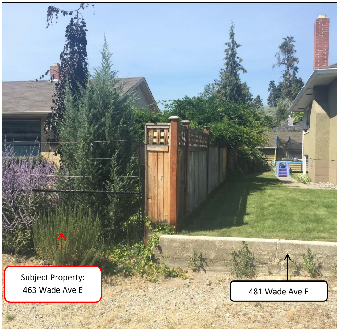
Figure 9 – Looking at property line between 463 Wade Ave E and 481 Wade Ave E
